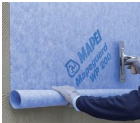
Instalace fólie Mapeguard WP 200
