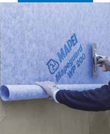
Instalace fólie Mapeguard WP 200
